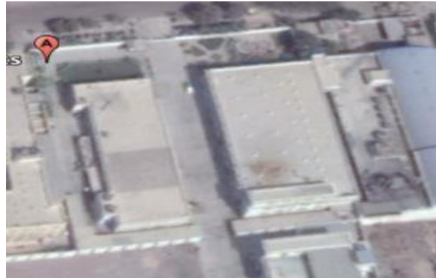
Figure 3: Plant Rooftop area
